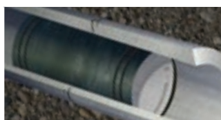
9. Deflate Packer & Remove it from the Pipe
